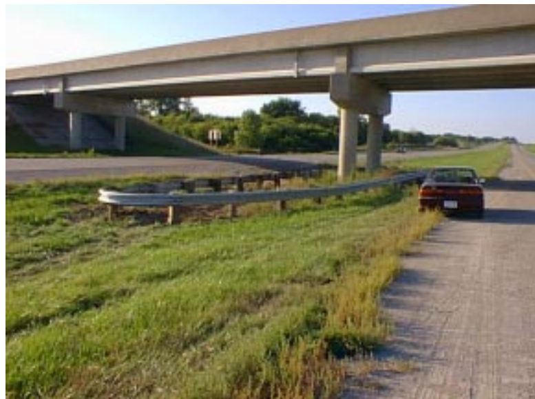
Figure 1. Typical bullnose median treatment around bridge piers.
