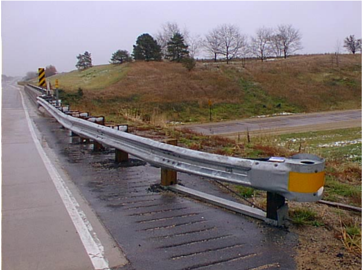
Figure 1. Modified Eccentric Loader Breakaway Cable Terminal
